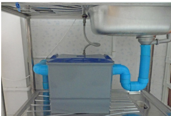
(a) Examples of grease traps Source: https://pantip.com/topic/35866812
